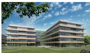
Banessa Business and Technology Park, Bucharest, Romania Design Office : Inginierii structurali Srl
