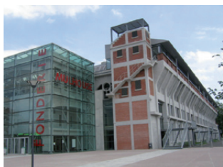
La Fonderie, University of Economic, Juridical and Social Sciences Design Office: Hagemüller Ingenieirie, Colmar Architecture Office: Morgiello - Pilsson / Emergence
